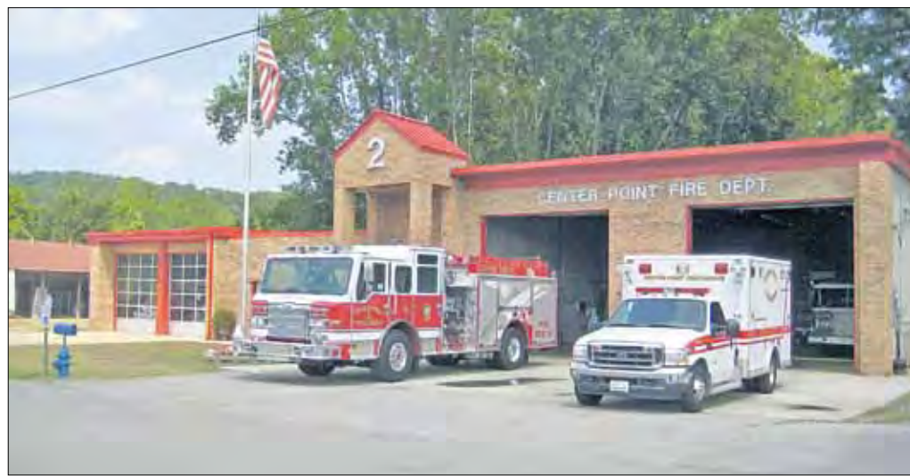
photo courtesy of Center Point Fire District
